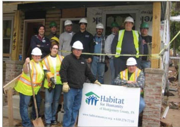
A group of volunteers from ABC member company Skanska USA Building, Inc. helped Habitat for Humanity build a duplex in Montgomery County, Pa.
